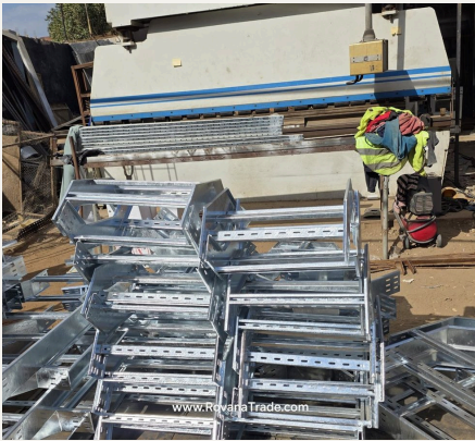
Ladder fittings formed in-house
