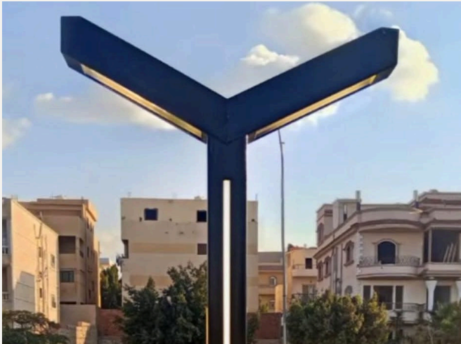
Square Y-arm with LED arms and a vertical light strip, installed
